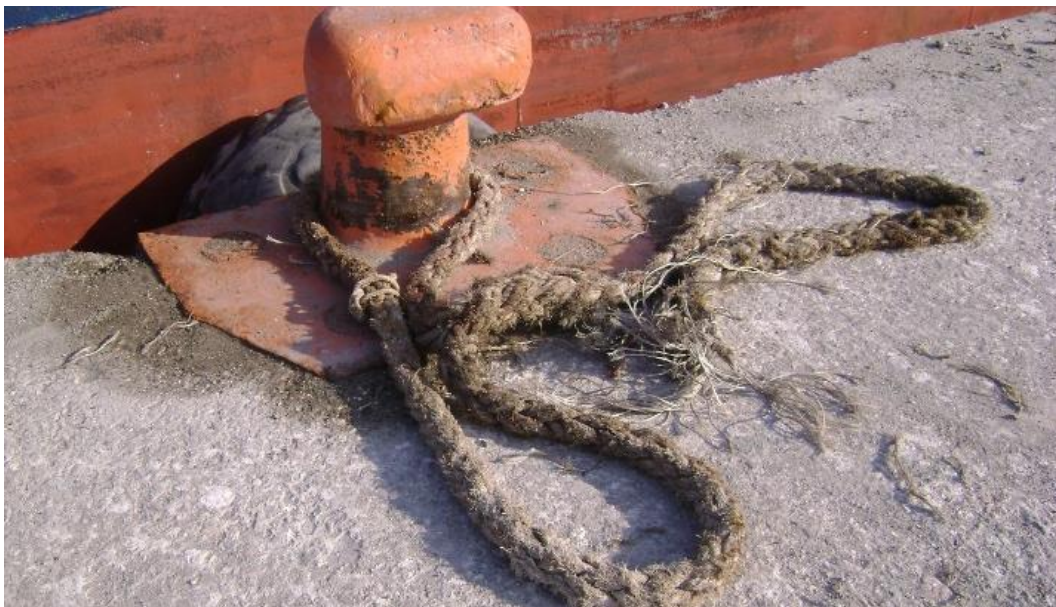
Image 6 The Part Of The Broken Rope Remaining On The Bollard
