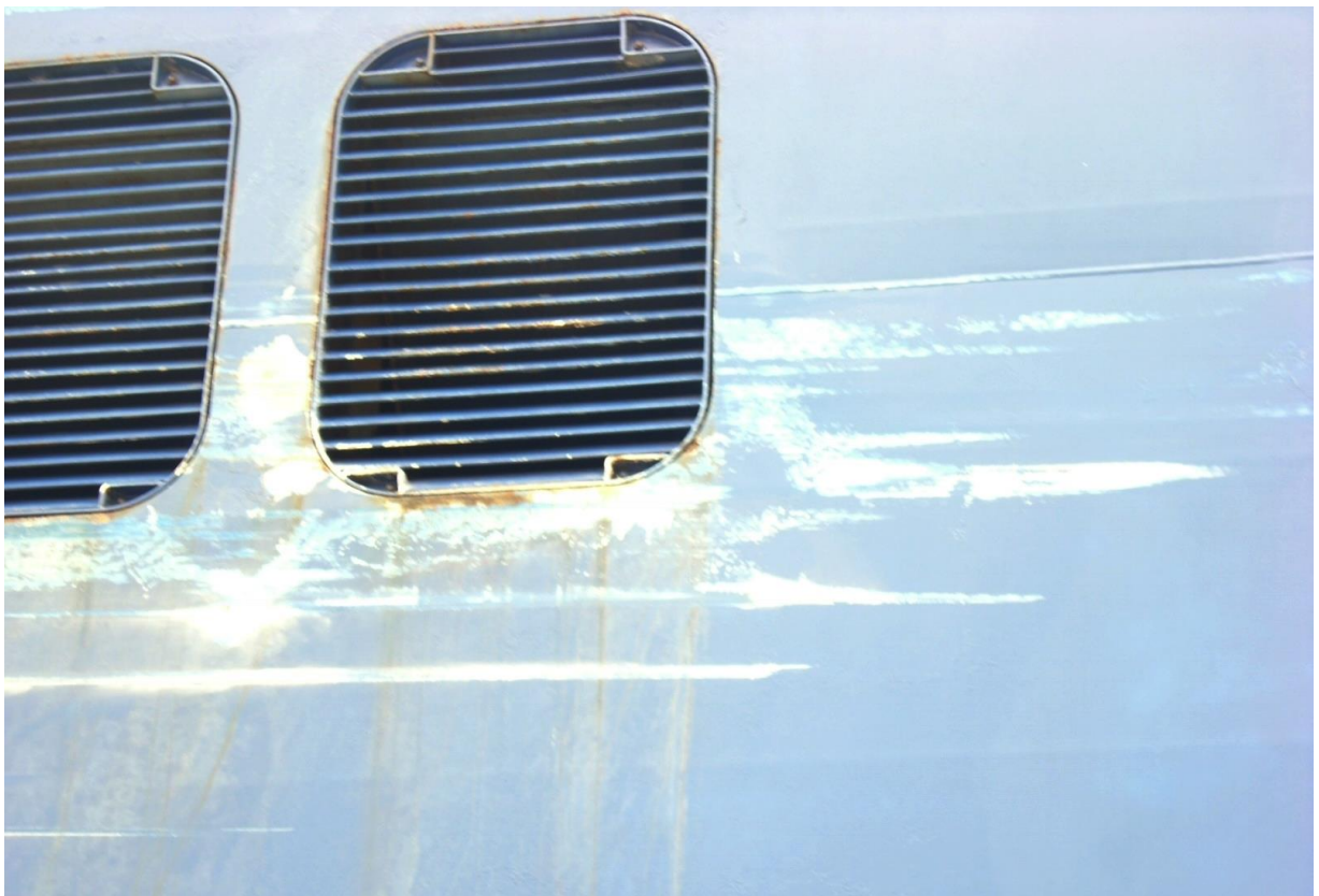
Figure 5: Damage to starboard stern of UND EGE
