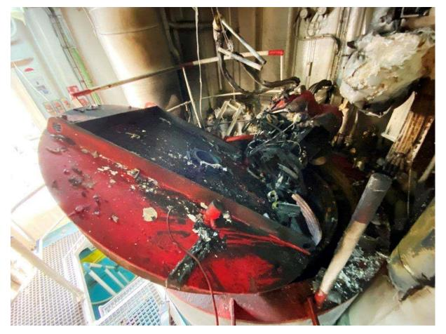
Image 7 Damage to Boiler Cover After Explosion
