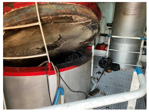
Image 8 Boiler Cover After Explosion
