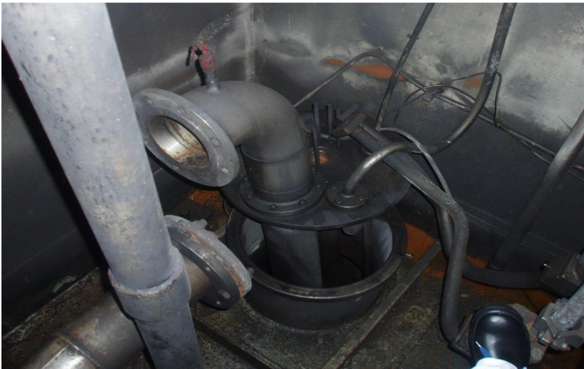
Figure 3: Cofferdam of No.2 Starboard Side Tank
