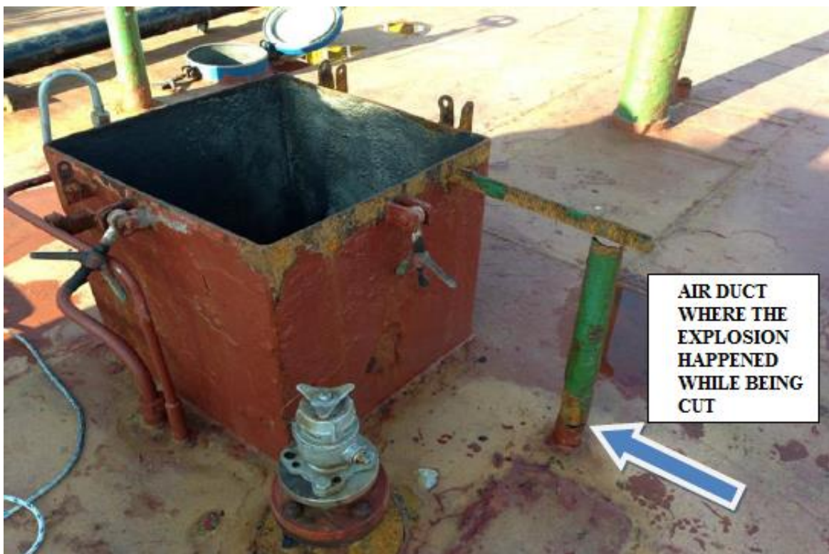
Figure 4: Entrance Manhole of the No.2 Starboard Side Tank Cofferdam
