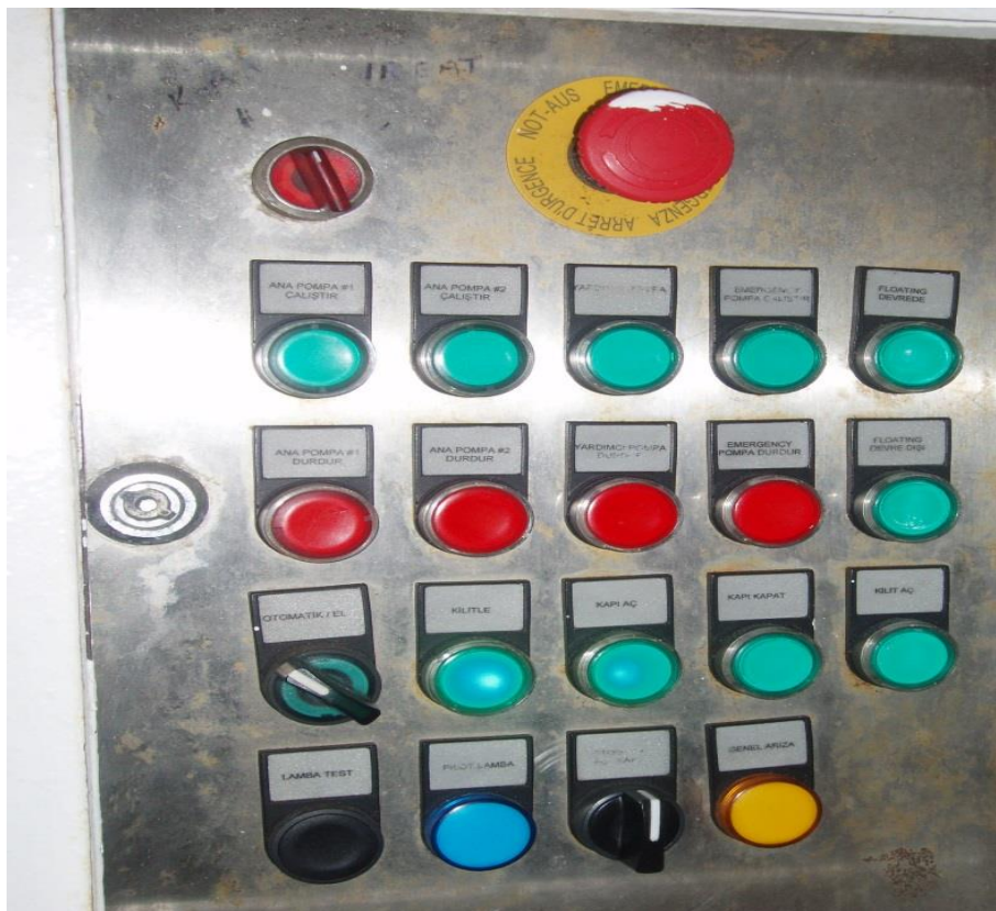
Picture 8 : Ramp Control Panel (Vehicle Deck)
