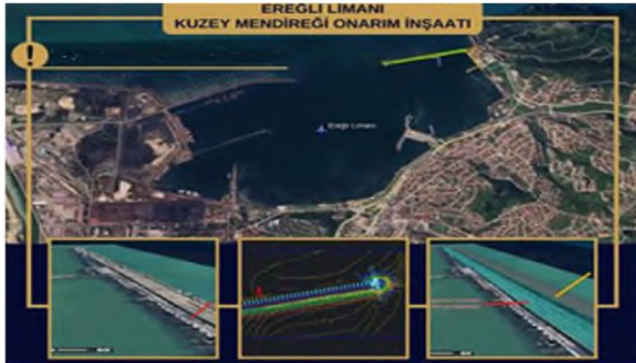
Image 25 Breakwater Repairs and Renovations
