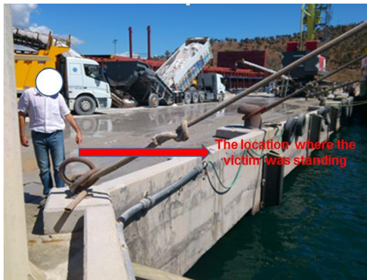
Picture 7: Dock No 4 where the accident occurred
