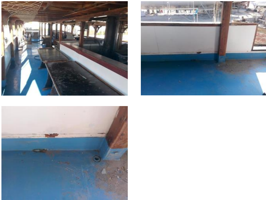
Figure 19: Passenger hall, bulwarks and the water drainage hole in front of the bulwarks
