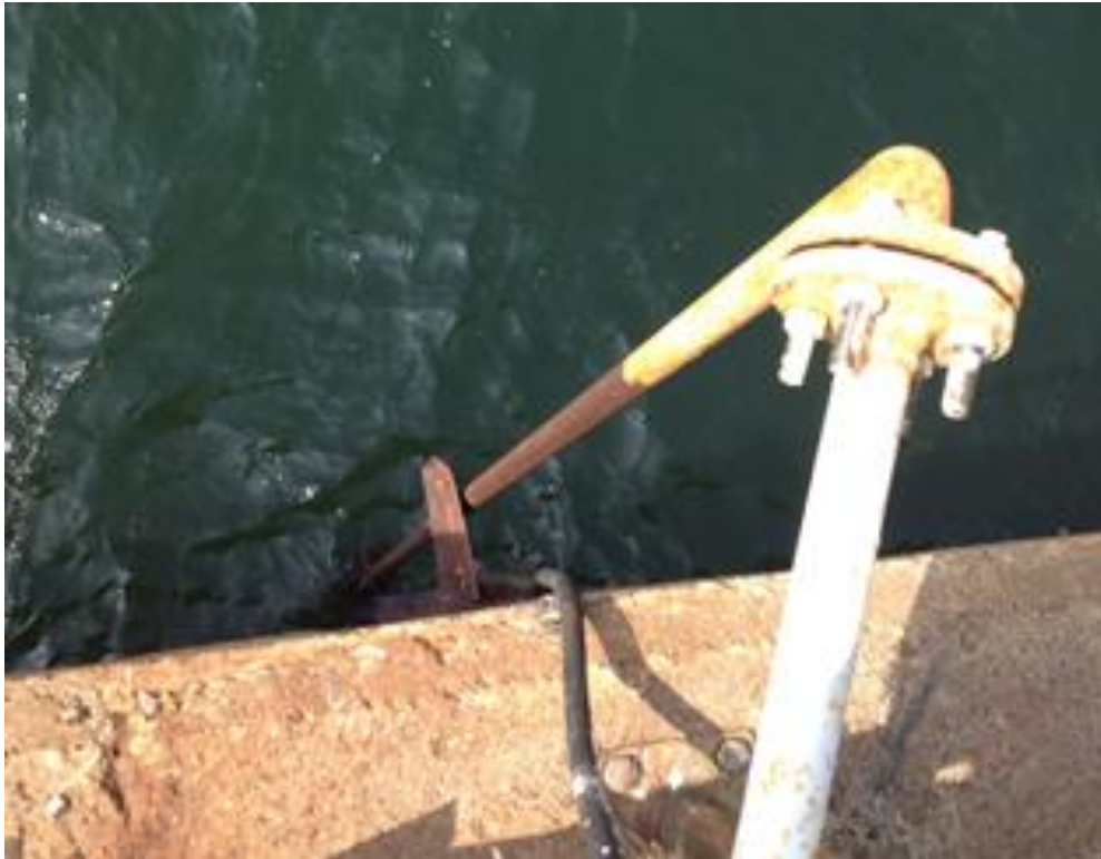
Figure 13: Gas Draining Line at the Platform
