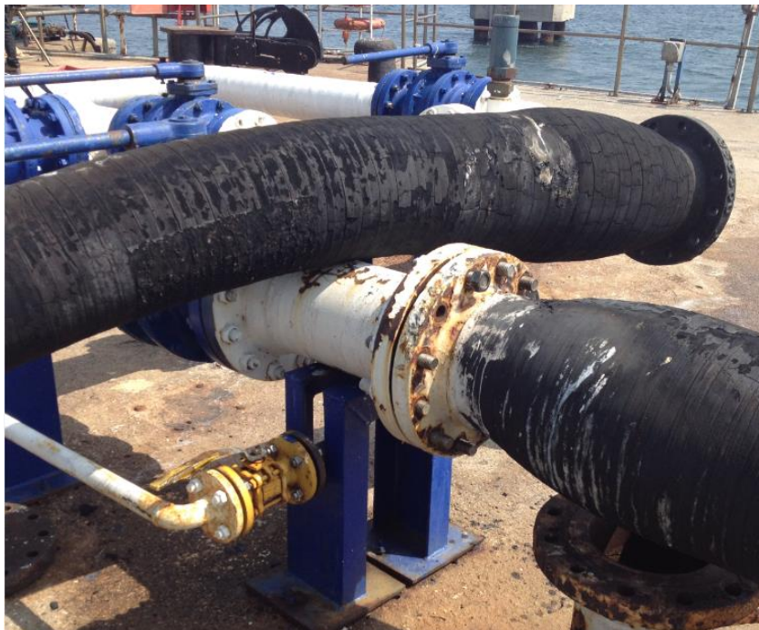
Figure 15: Hose used in the Cargo Operation
