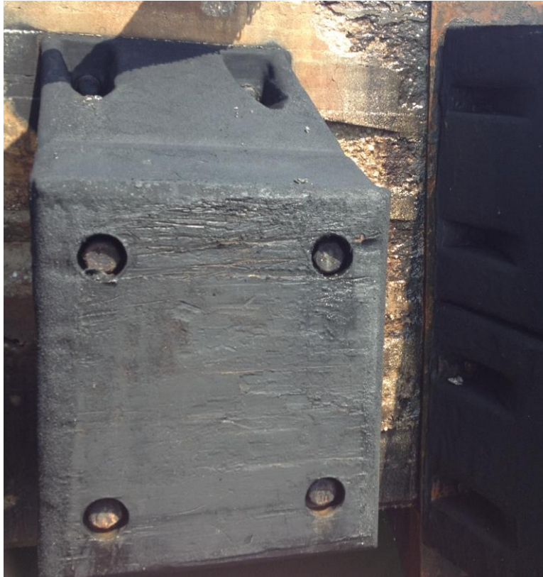
Figure 8: Platform Fender Damaged by the Fire
