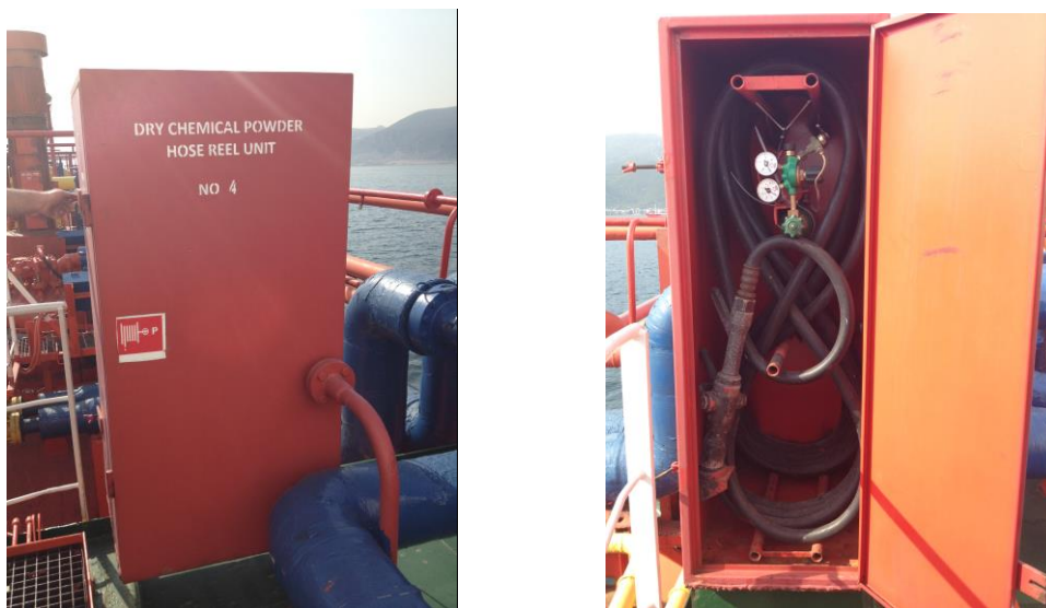
Figure 24,25: Fixed Dry Chemical Powder Firefighting System
