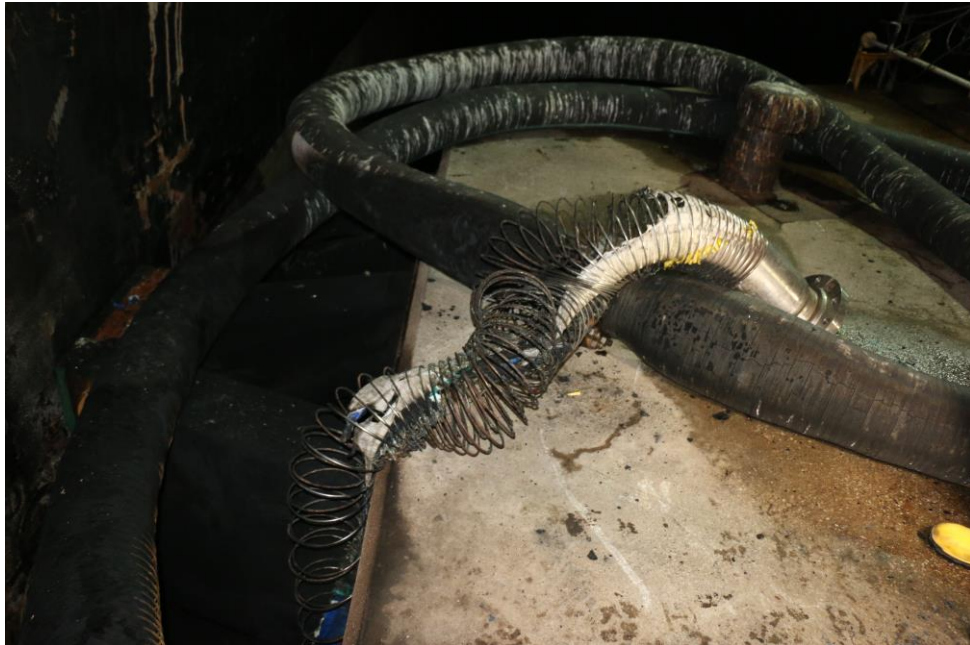
Figure 18: Hose used in Releasing Gas Vapor Remaining in the Tanks into the Sea.
