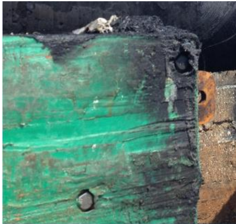
Figure 9: Platform Fender Damaged by the Fire
