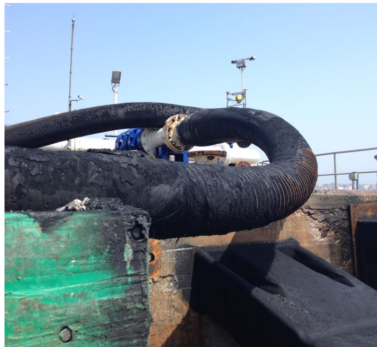
Figure 7: Black Hose Damaged by the Fire
