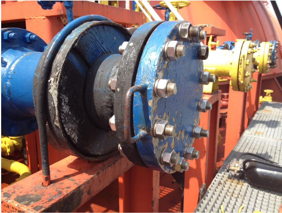
Figure 19: The Vessel's Manifold
