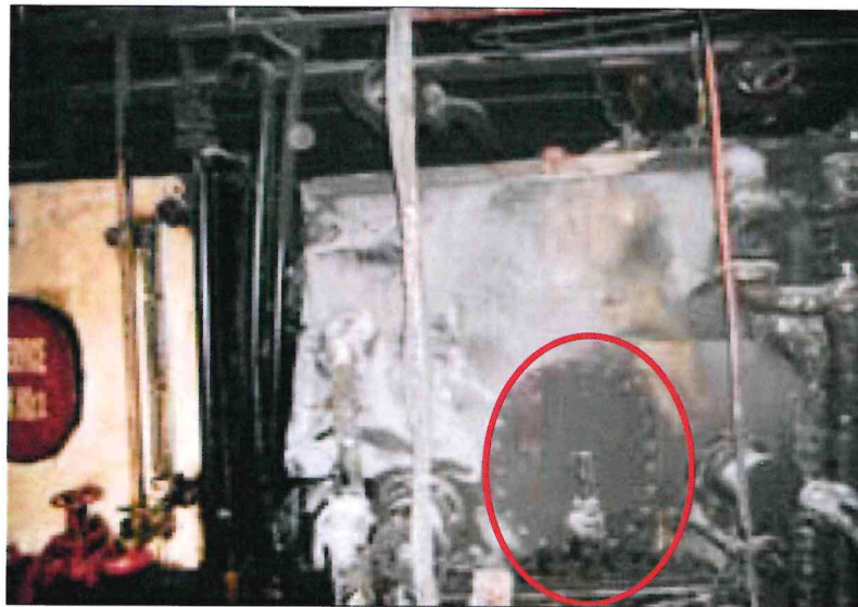
Image 8 Condition of Fuel-Oil Service Tank After the Explosion
