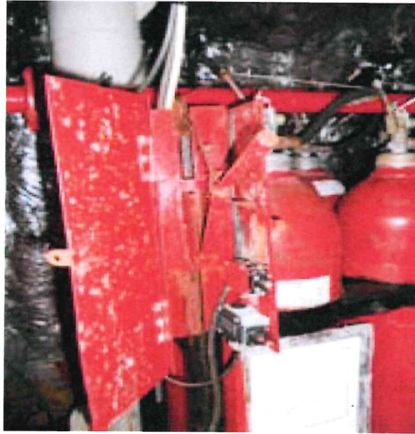
Image 9 CO 2 Detonation Mechanism
