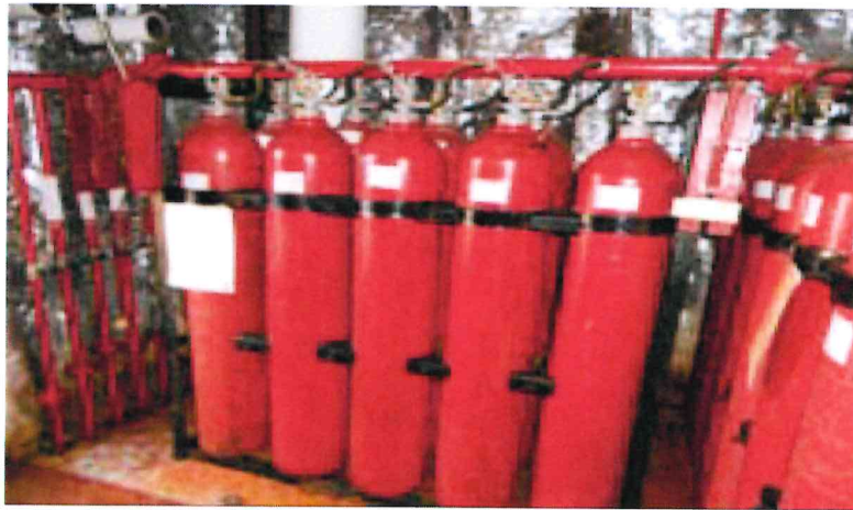
Image 10 CO 2 Cylinders Reserved for the Engine Room
