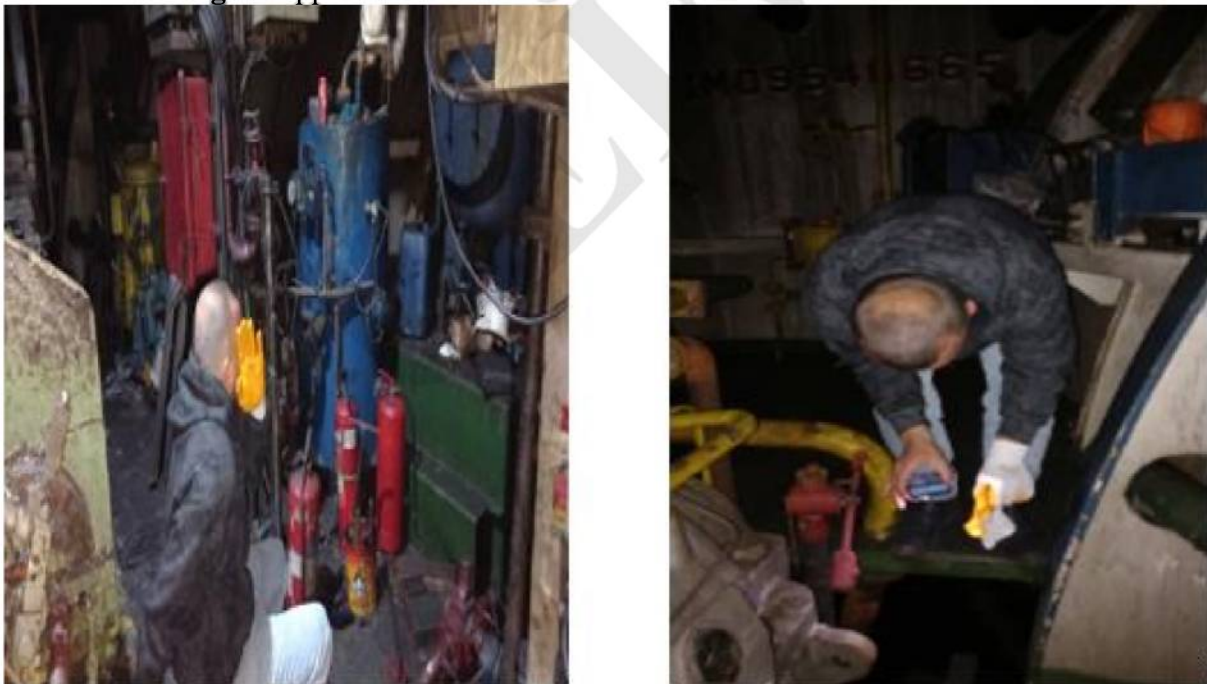
Image 6 Approximate locations of the deceased subcontractor workers
